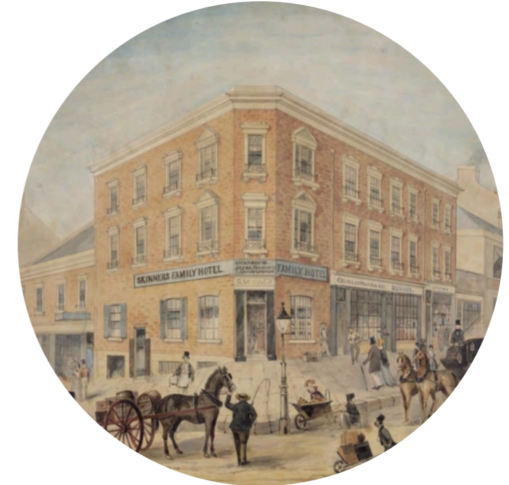
28. Watercolour drawing of Skinner's Family Hotel, 1849. The Former Skinner's Hotel is located at the George and Hunter st within the site boundary. The drawing shows the hotel in face brick with rendered window dressings. It more clearly illustrates a basement level to Hunter st.
